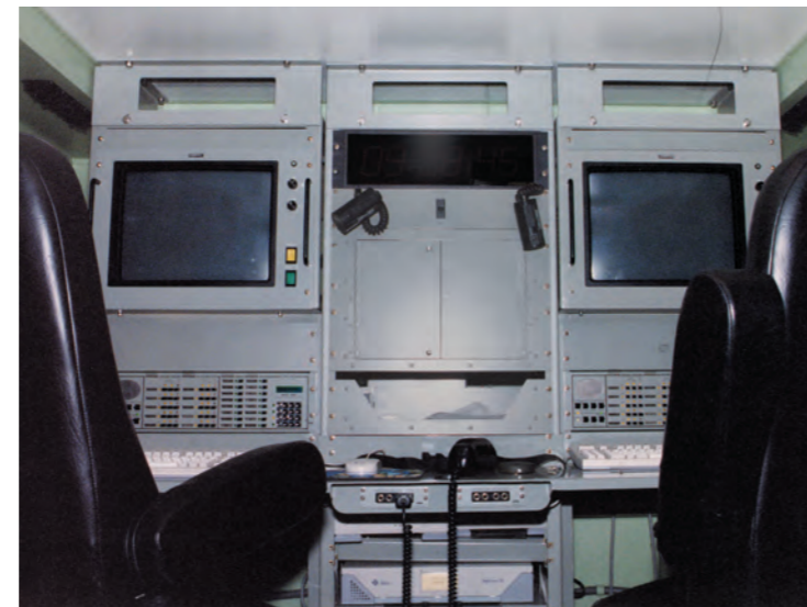
Two controller consoles
