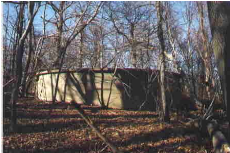
The picture above is the actual water supply that fed the entire base And heated each building. It is no longer used now since the base first closed in 1959.
