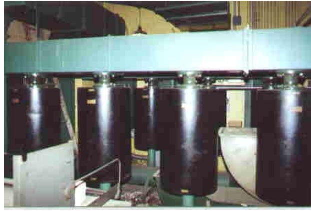
Giant air tanks provided a constant air supply to the operations building or “Bombproof” building
